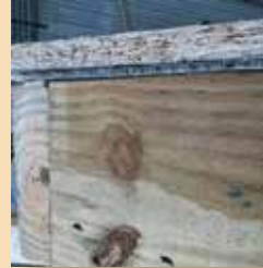
Floor Installation R6
