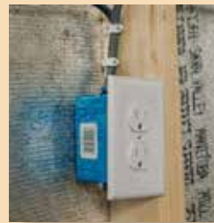
Tamper Proof or GFCI Receptical
