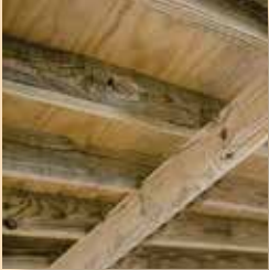
12" On-Center Floor Joists
