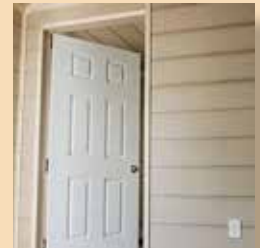
Interior Wall (Cottage)
